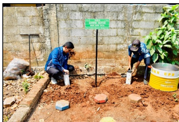
Gambar 8. Praktik Proses Pemasangan Pipa Casing Biopori
